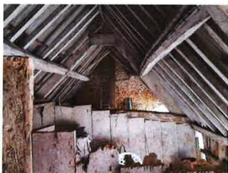
Boarding is not evident under each tie beam and is not historic in nature
